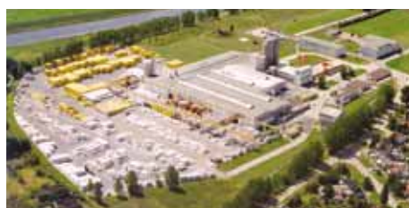
Calbe Factory, Germany
